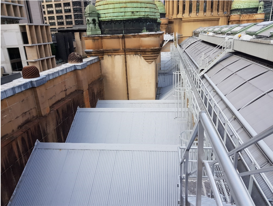
Figure 11: Typical New Access Walkways
