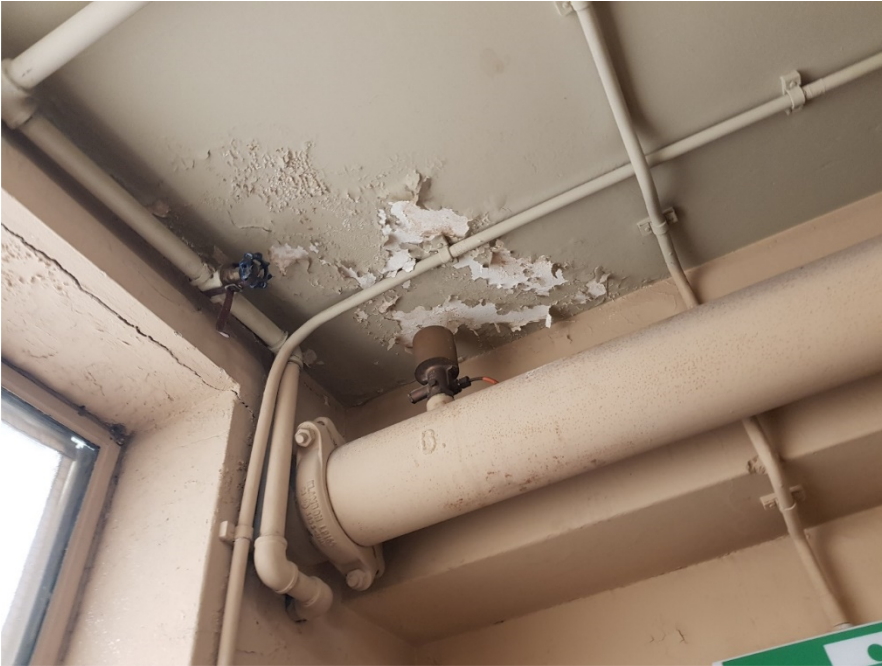
Figure 29: Spalling Concrete
