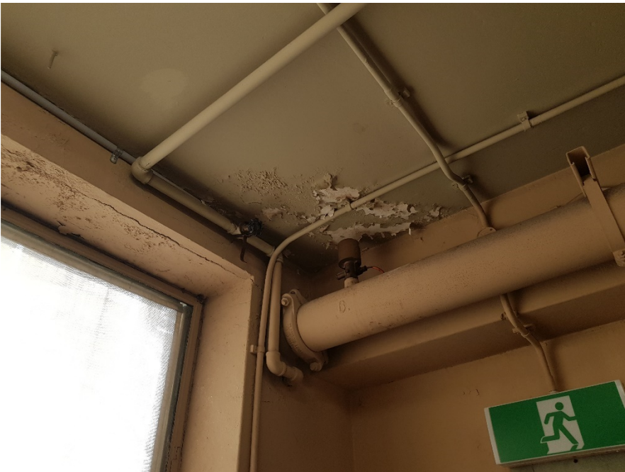
Figure 25: Cracking in Lintel
